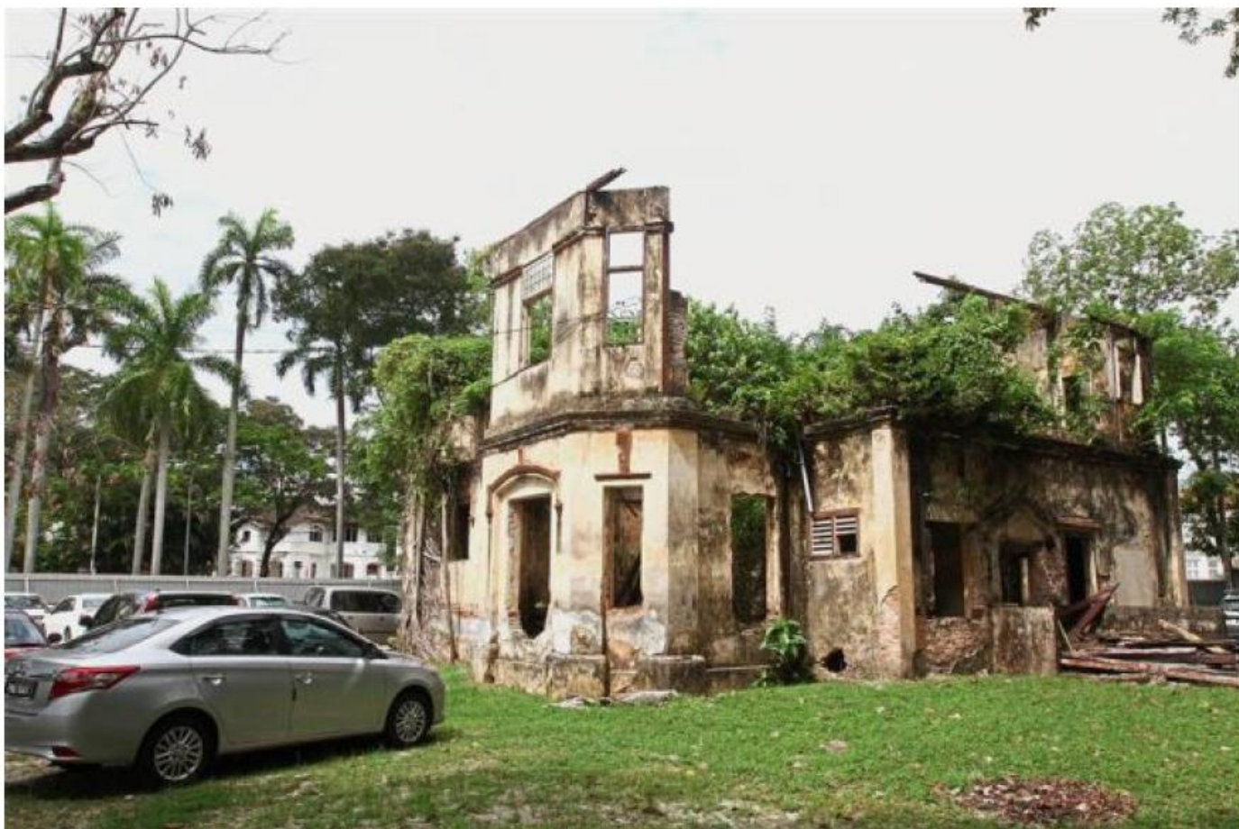
Controversial project: The heritage building was torn down last year to make way for the IMC.
